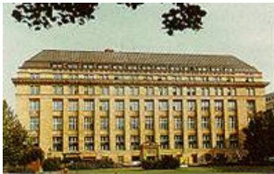
National Bank Austria 5.000 optical ports
